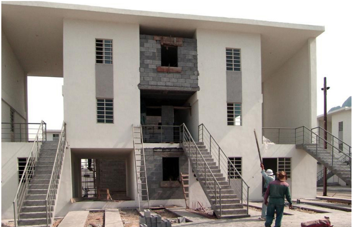
Figure 2: Monterrey Houses — Monterrey, Mexico by Elemental, showing the ease with which the structure is repaired or added to by, and at the will of the homeowner.
